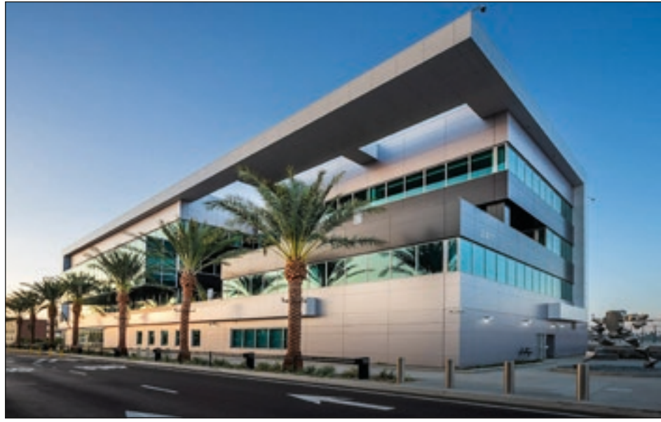
Sundt construction has finished a new administration building at San Diego International Airport. Photo courtesy of San Diego International Airport
